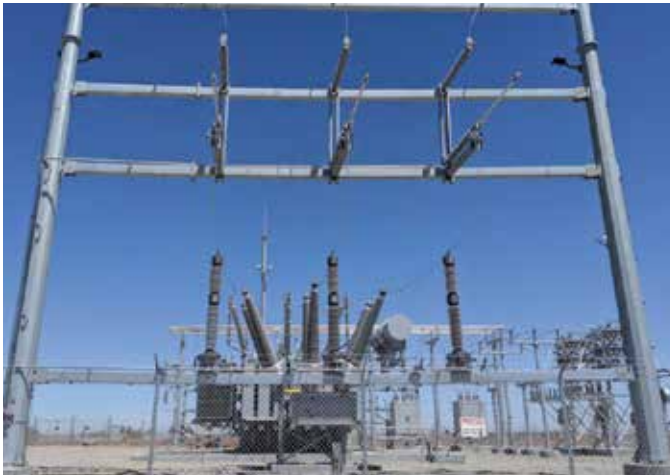
Mount Signal 2 Solar | CA | 165 MVA, 34.5/230kV
