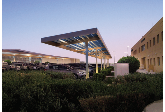
Qatar Science & Technology Park | Doha, Qatar | 700kW
