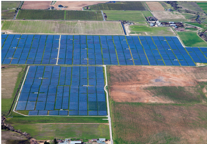
SMUD: McKenzie, Kammerer, Bruceville, and Dillard | 69MW
