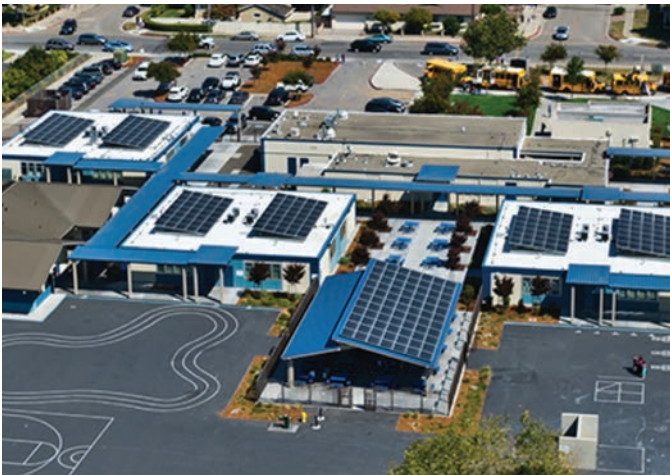
San Jose Unified School District | 13 schools, CA | 7.2MW
