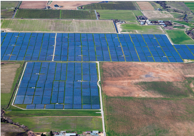
SMUD: McKenzie, Kammerer, Bruceville, and Dillard | 69MW
