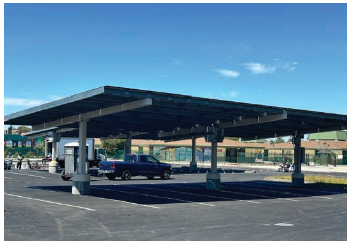
Franklin-McKinley School District, CA | 2.74MW
