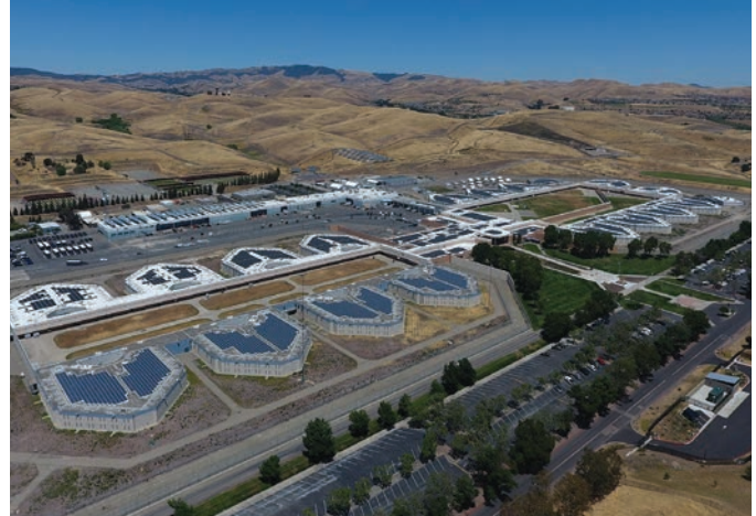
SMUD | McKenzie, Kammerer, Bruceville, and Dillard | 69MW
