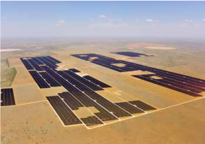
Prospero 1 & 2 | Andrews, Texas | 550MW
