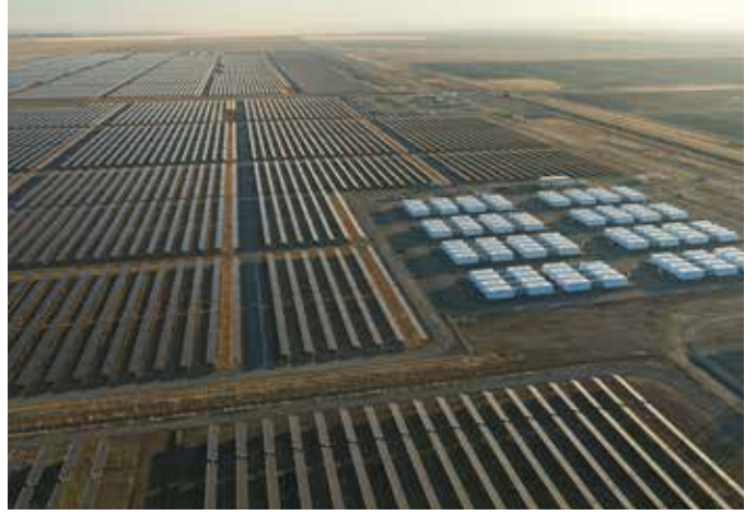
Solar Blue | Stratford, California | 250MW
