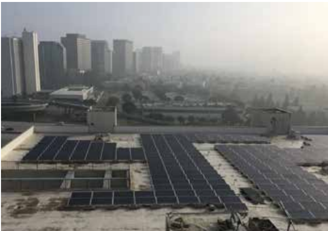
U.S. Veterans Administration Hospital | FL and CA | 5.7MW
