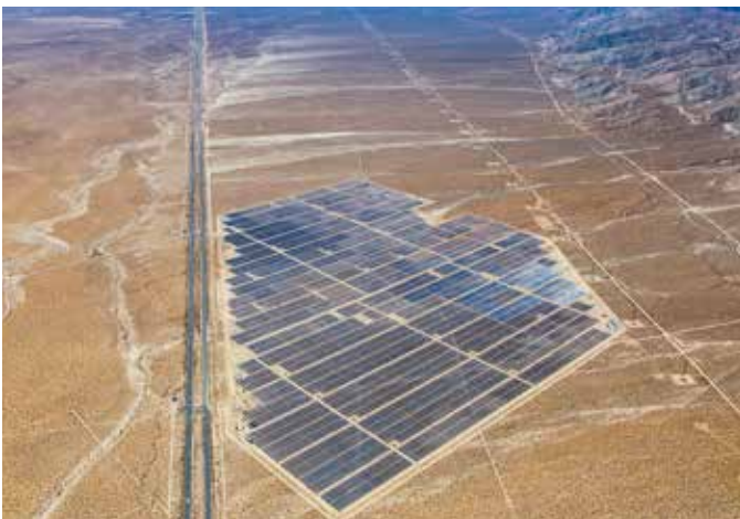
RE Barren Ridge | Kern County, CA | 60MW
