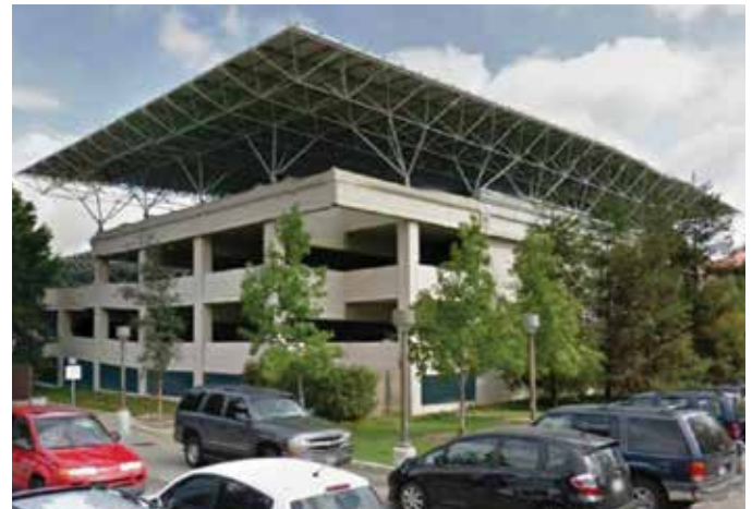
California Institute of Technology | Pasadena, CA | 1.4MW
