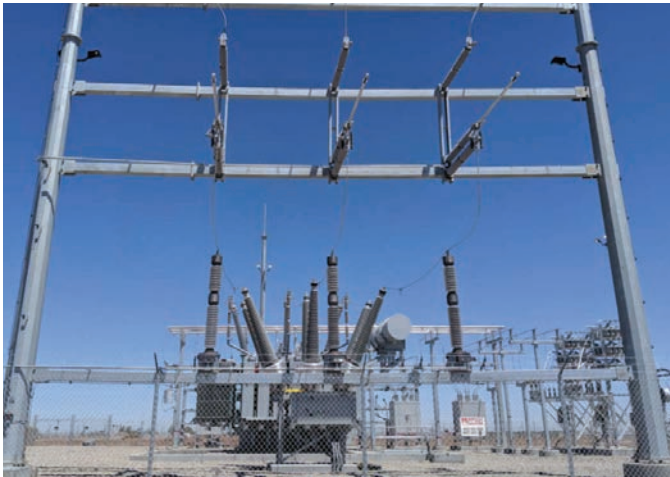
Mount Signal 2 Solar | CA | 165 MVA, 34.5/230kV
