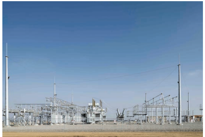
Aquamarine | Stratford, CA | 34.5/230kV and 320MVA
