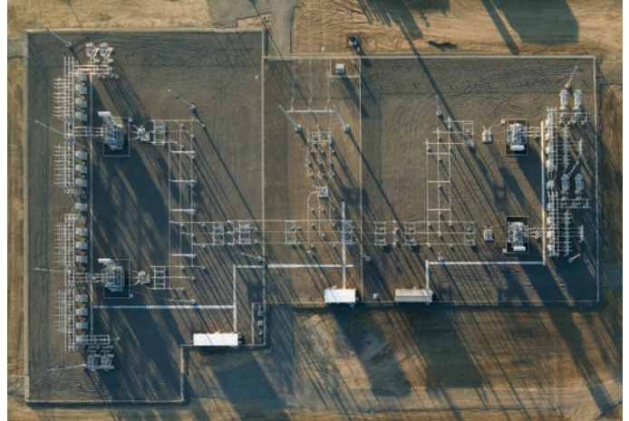
Solar Blue | Stratford, California | 34.5/230kV, 250MVA
