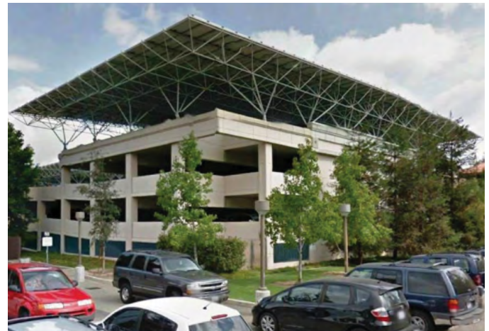
California Institute of Technology | Pasadena, CA | 1.4MW
