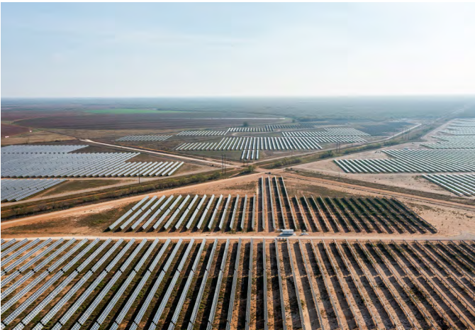
Elara Solar | Pearsall, Texas | 130MW
