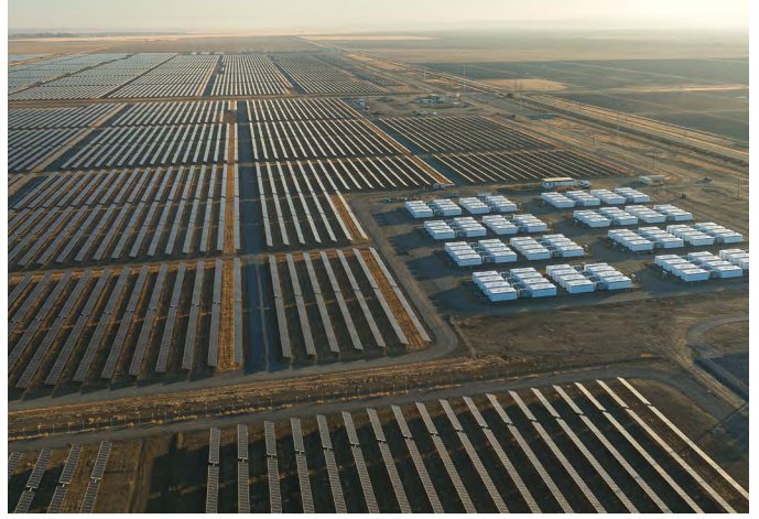
Solar Blue | Stratford, California | 250MW
