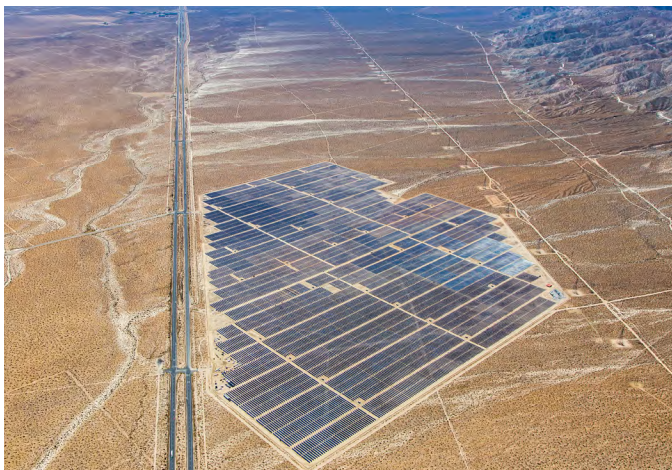
RE Barren Ridge | Kern County, CA | 60MW
