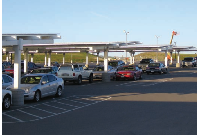
Lancaster Unified School District | 23 schools, CA | 5.5MW
