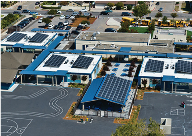
San Jose Unified School District | California 7.2 MW Solar | 13 schools
