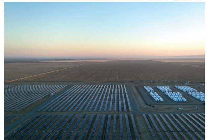
Chestnut | Kings County, California 135 MW Energy Storage | 150 MW Solar
