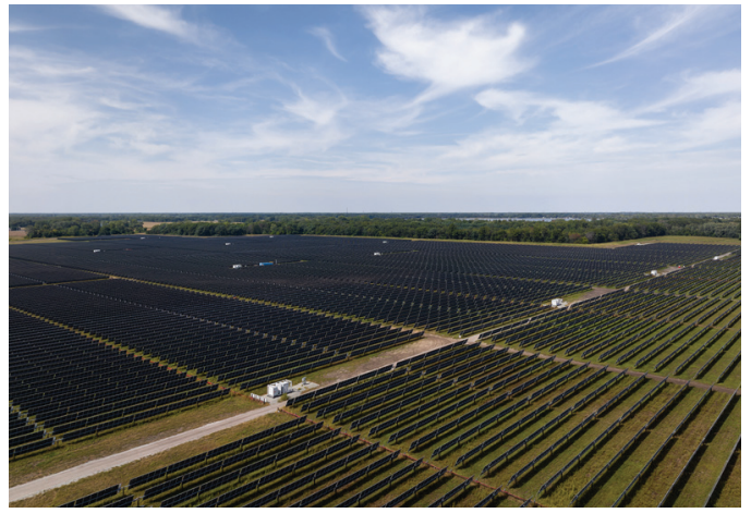
Mammoth North | Monterey, Indiana 400 MW Solar
