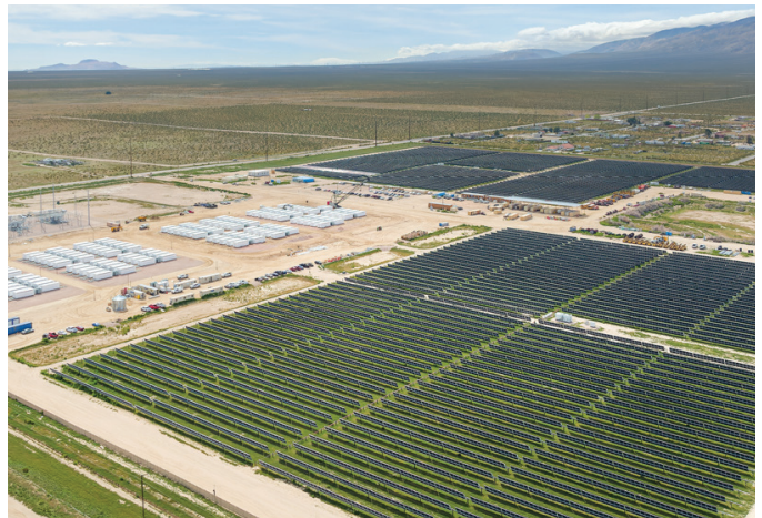
Eland | California City, California 200 MW Solar
