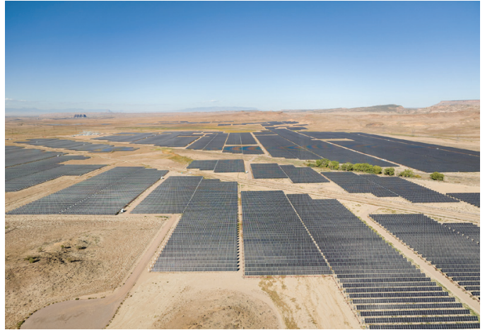
San Juan | Kirtland, New Mexico 200 MW Solar | 400 MWh Energy Storage
