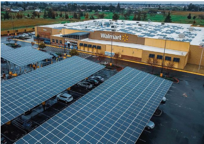
Walmart | 7 locations | Central California 2.8 MW Solar
