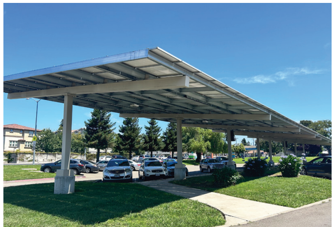
Hayward Unified School District | California 5.3 MW Solar | 33 schools
