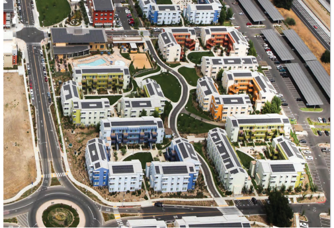
UC Davis West Village | Davis, California 340 kW Solar
