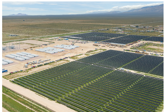
Eland | California City, California 200 MW Solar
