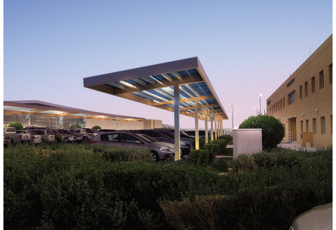
Qatar Science & Technology Park Doha, Qatar | 700 kW Solar
