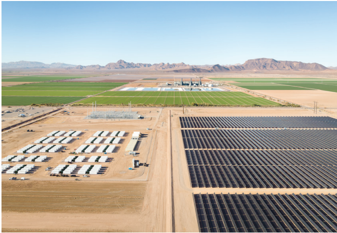
Harquahala | Tonopah, Arizona 1.2 GWh Energy Storage | 450 MW Solar
