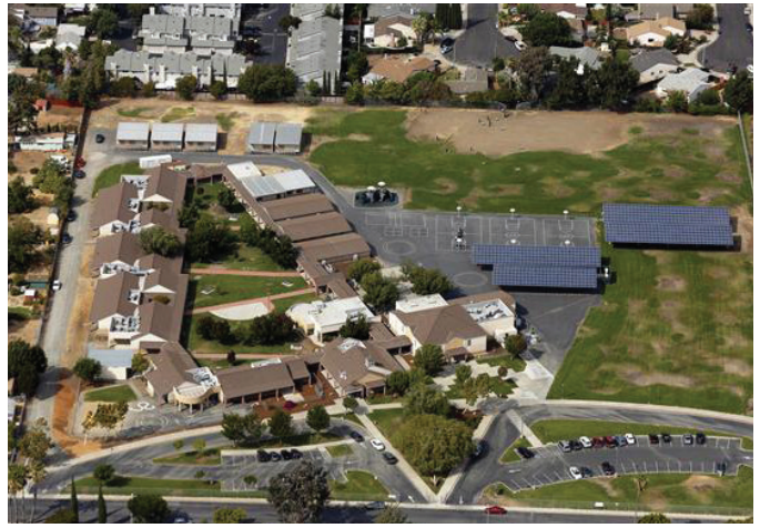
Pittsburg Unified School District | California 4 MW Solar | 13 schools
