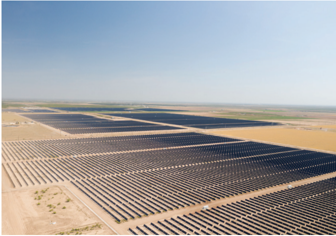
Taygete 1 & 2 | Pecos County, Texas 500 MW Solar
