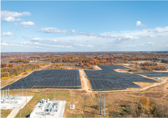
River Fork | Albion, Michigan 149 MW Solar | 34.5/138 kV Substation
