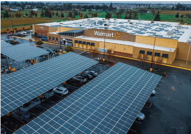
Walmart | 7 locations | Central California 2.8 MW Solar
