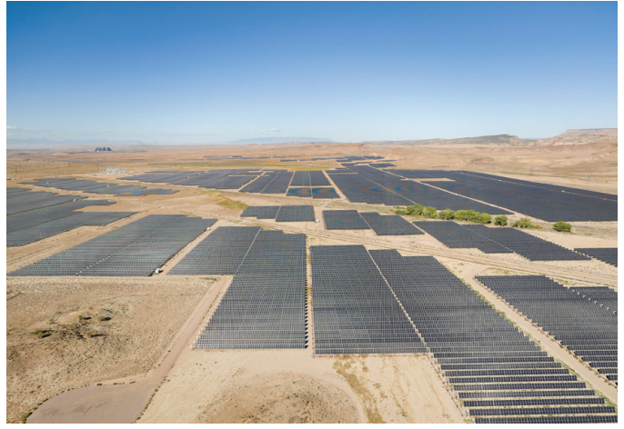
San Juan | Kirtland, New Mexico 200 MW Solar | 400 MWh Energy Storage
