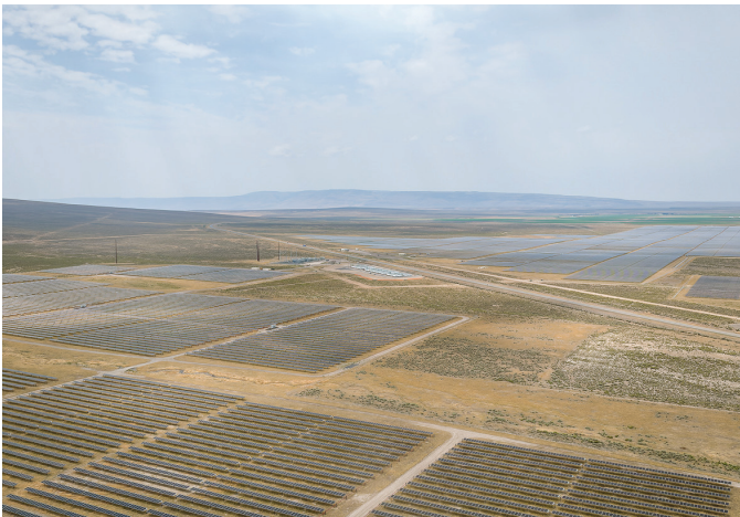
Franklin Solar | Rogerson, Idaho 100 MW Solar | 240 MWh Energy Storage
