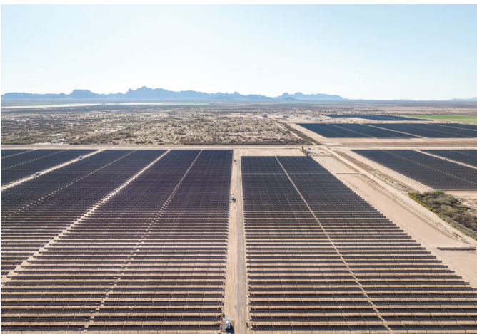
Harquahala | Tonopah, Arizona 450 MW Solar | 1.2 GWh Energy Storage
