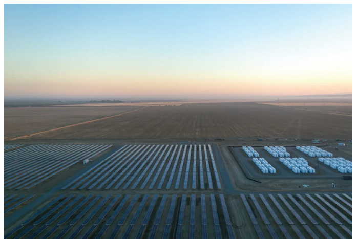
Chestnut | Kings County, California 230 kV, 200 MVA Substation 150 MW Solar | 135 MW Energy Storage
